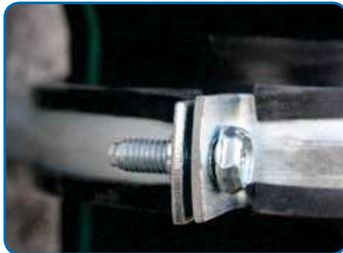
Figure 5 - Incorrect tightening:
