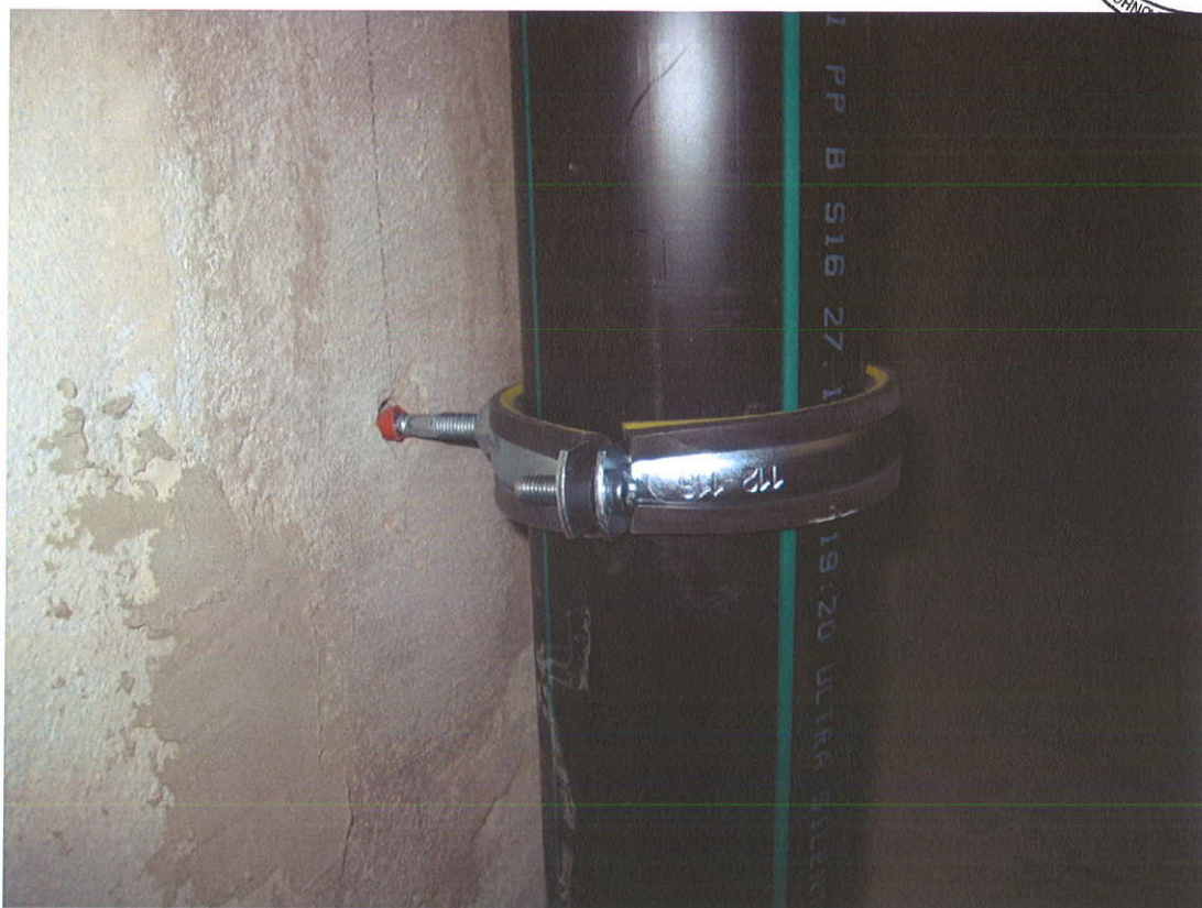
Figure 5 Waste water system "Ultra Silent 110 x 3.4" with pipe clamps "Müpro yellow, with spacer 5 mm".
